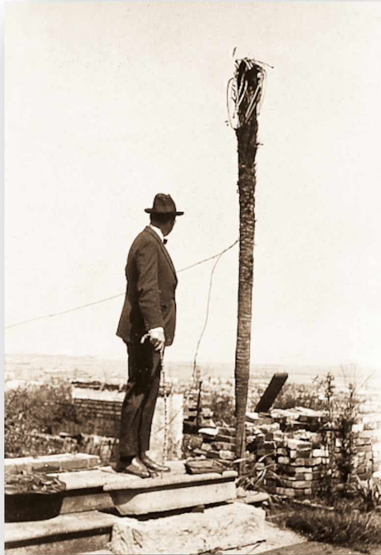
Sydney Bruce views the ruins of 203 Bluff Rd S of Yokohama beyond.
